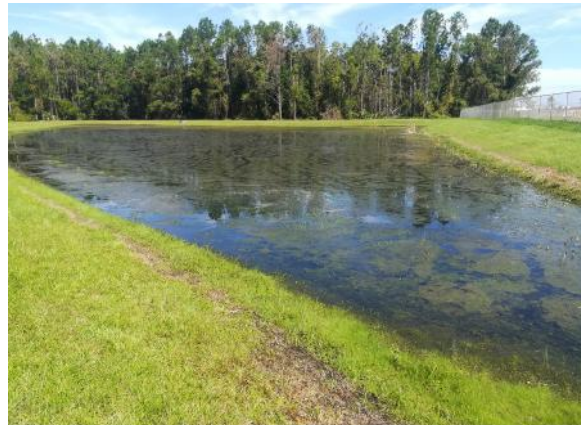
Pond #1: Treated shoreline grasses and submersed weeds.
